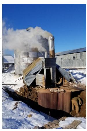
sheds so the heat would be pulled into the shed and into the bin blower fan. I set it up so the smoke had to go through the trench. The mud under this area was about the perfect mix of clay and sand for using in a rocket stove. The mud was well worked into a soft consistency after our running around there and perfect for sealing the trench, chimney, and connecting pipes. And so my 'rocket' stove was complete with very little outside inputs.
